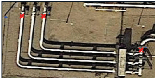
Leak locations confirmed
