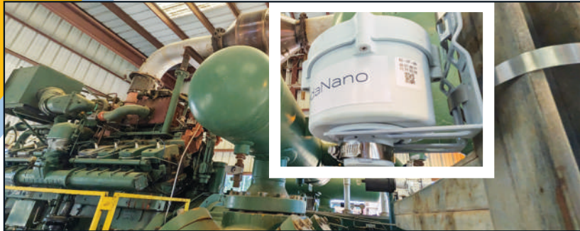
MethaneTrack™ endpoint mounted on tank near compressor
